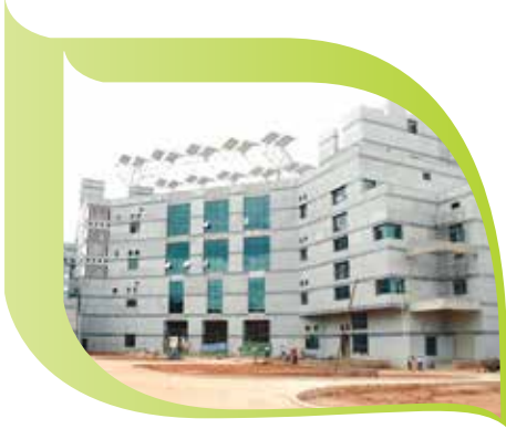
Instem building - NCBS campus
